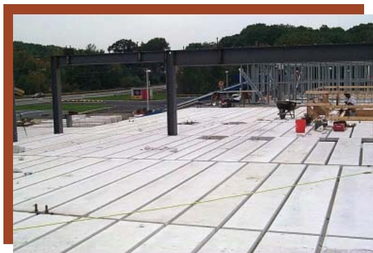
Marriott Hotel, Lincoln, RI: AAC Floor Panels Supported on Light Gauge Metal and Steel Framing (Photo by Dewberry)
