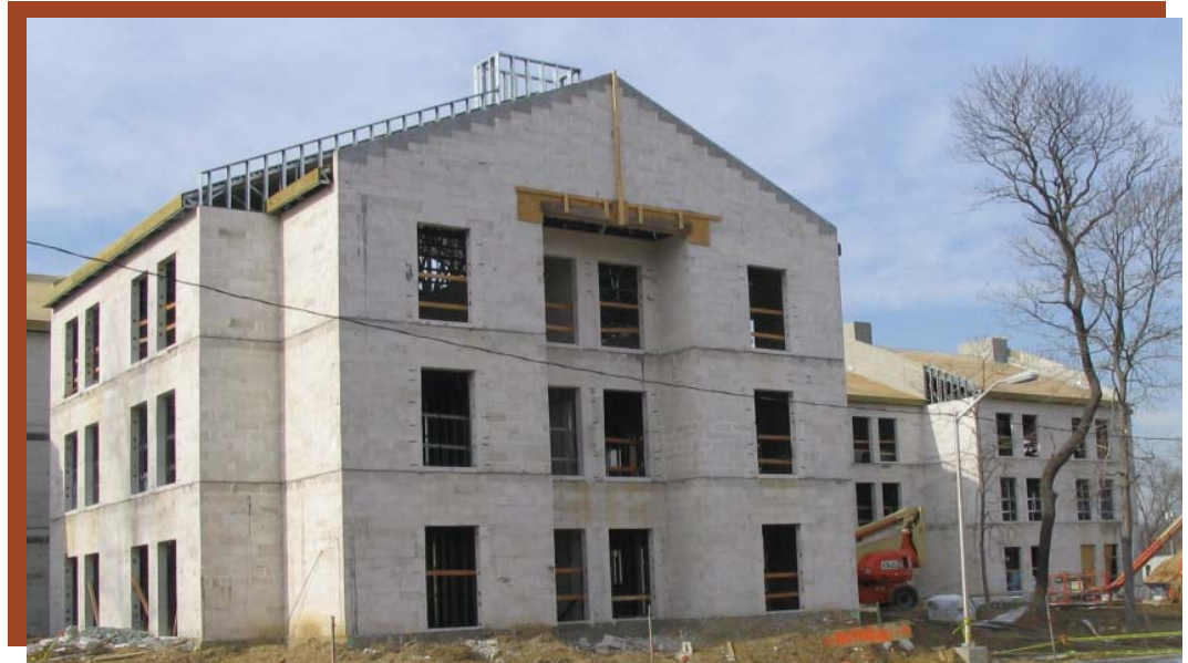
SUNY at Stony Brook Graduate Apartments: AAC Masonry Walls and Precast Hollow Core Floors. (Photo by Dewberry)
