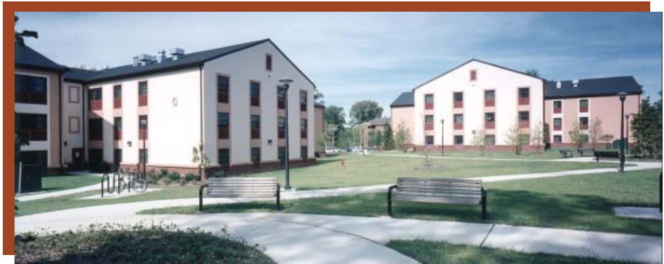
SUNY at Stony Brook Undergraduate Apartments: AAC Floor and Wall Panel Construction (Photo by Bob Zucker)
